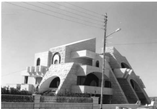
Fig. 5. Villa, Arch. Waddah Alabedi
